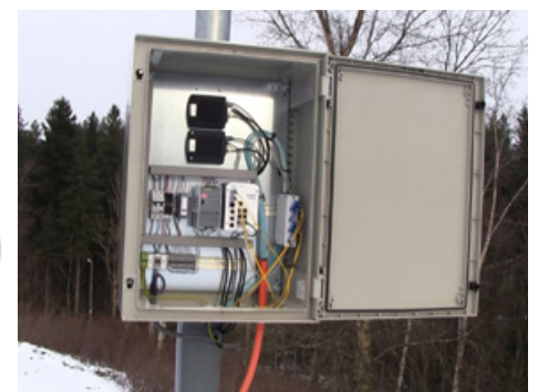
The live footage from the thermal imaging cameras is encoded and transported to the control station through fiber optic cables.
